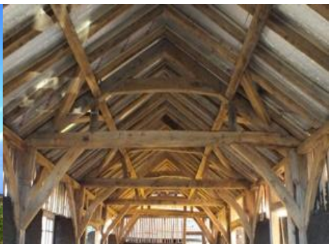
The Mud and Stud barn
